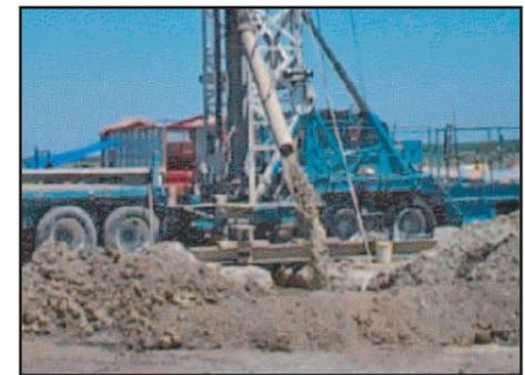
Figure 3. Reverse rotary drill rig re-circulating drilling fluid into pit.
